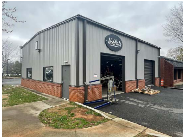
1,800 SF Mechanical Garage
