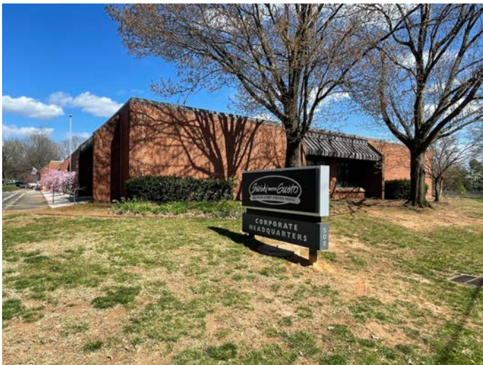
Structural Steel + Brick Construction
