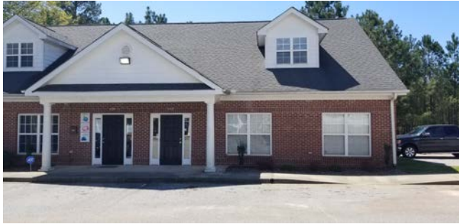
Front of Building
